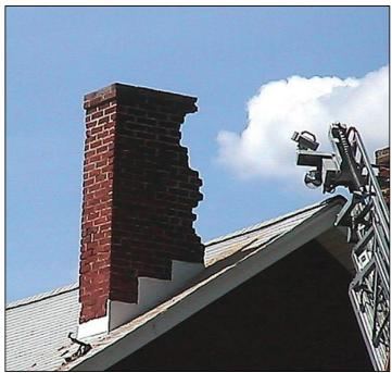
Figure 4.3.4.3.1: Chimney Damage (Fayetteville, PA) - Aug 2011 Earthquake<sup>35</sup>
