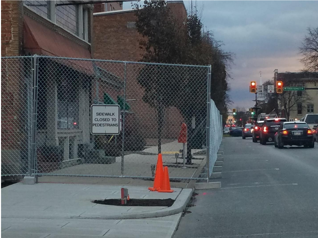
Sidewalk in front of 56 N Main Street, Chambersburg.
