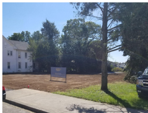
Project Site - Post-demolition - Fall 2021
