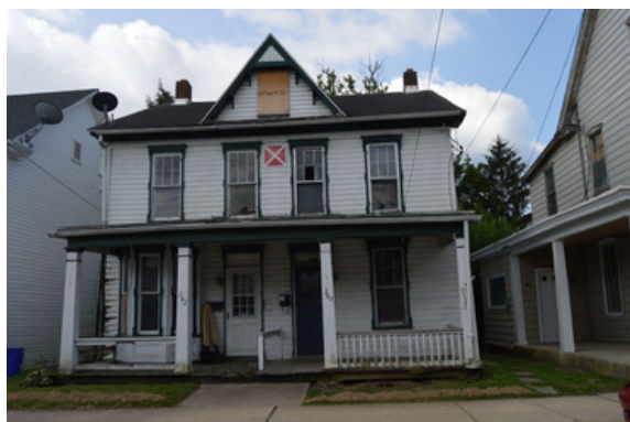
242-244 W. 2nd Street - Pre-demolition
