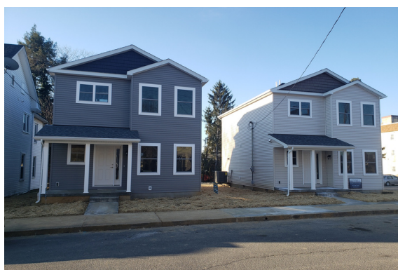
Project Site - Post-construction - December 2022
