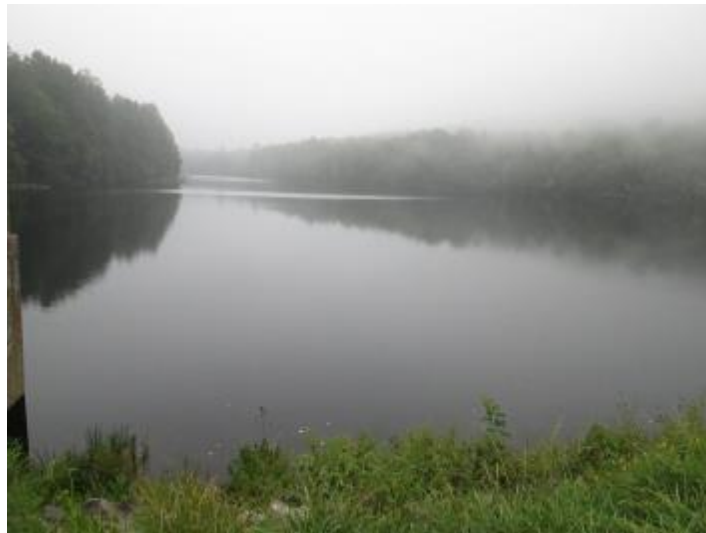
Figure 3.1.2.5.12: Antietam Dam Entrapment Area
