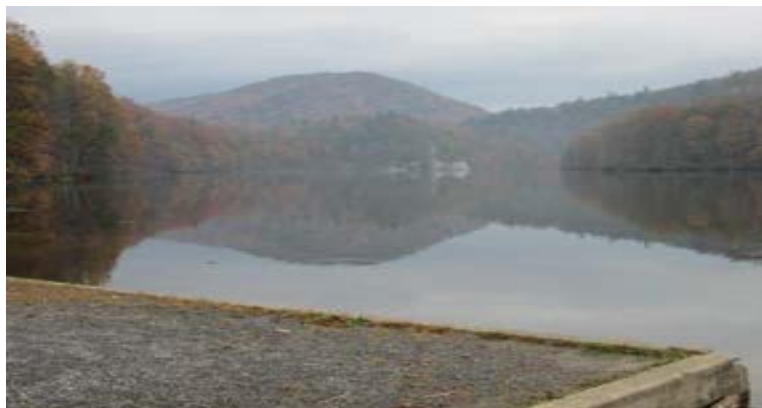
Figure 3.1.2.5.6: Entrapment Area of the Roxbury Dam
