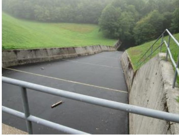
Figure 3.1.2.5.13: Antietam Dam Spillway
