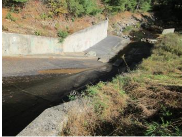
Figure 3.1.2.5.17: Carbaugh Run Dam Spillway
