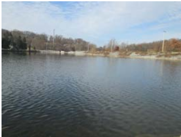
Figure 3.1.2.5.30: Lower Lake Royer Dam Wall
