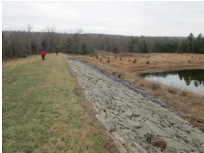
Figure 3.1.2.5.26: Meadow Grounds Dam Wall
