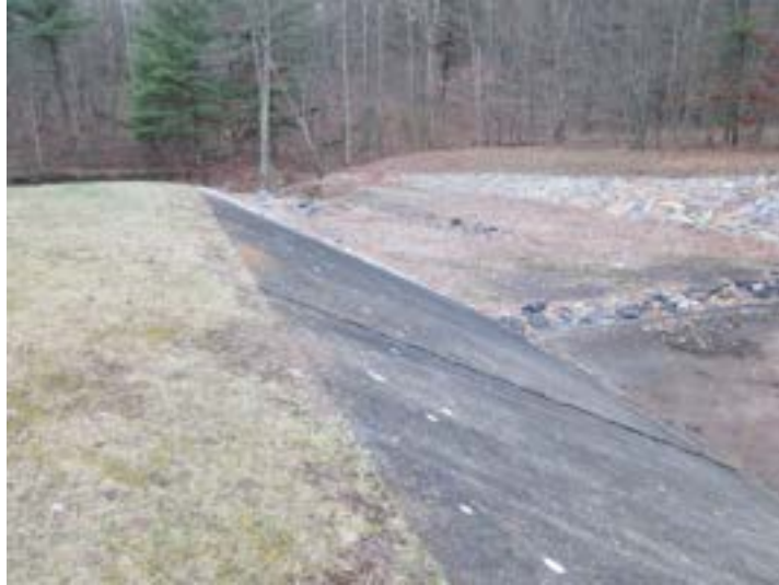
Figure 3.1.2.5.25: Meadow Grounds Dam Spillway
