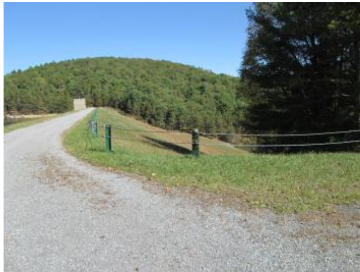
Figure 3.1.2.5.22: Long Pine Run Dam Wall
