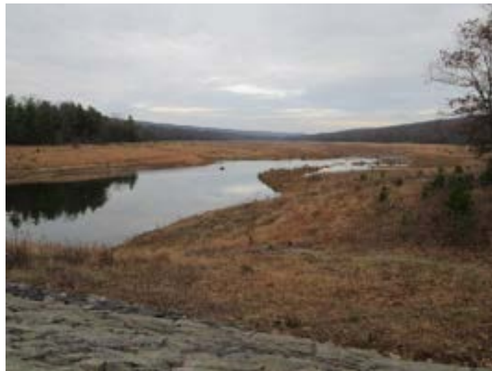
Figure 3.1.2.5.24: Meadow Grounds Dam Entrapment Area
