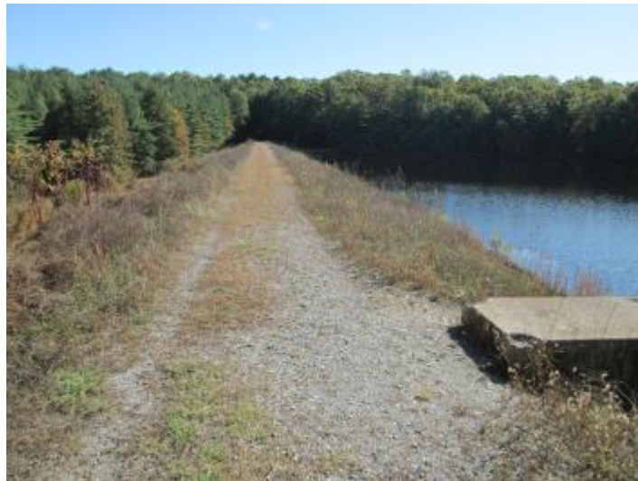
Figure 3.1.2.5.18: Carbaugh Run Dam Wall
