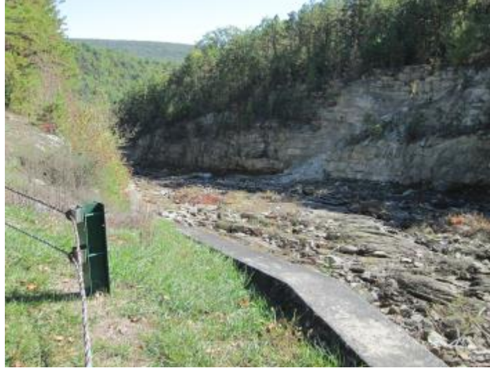
Figure 3.1.2.5.21: Long Pine Run Dam Spillway
