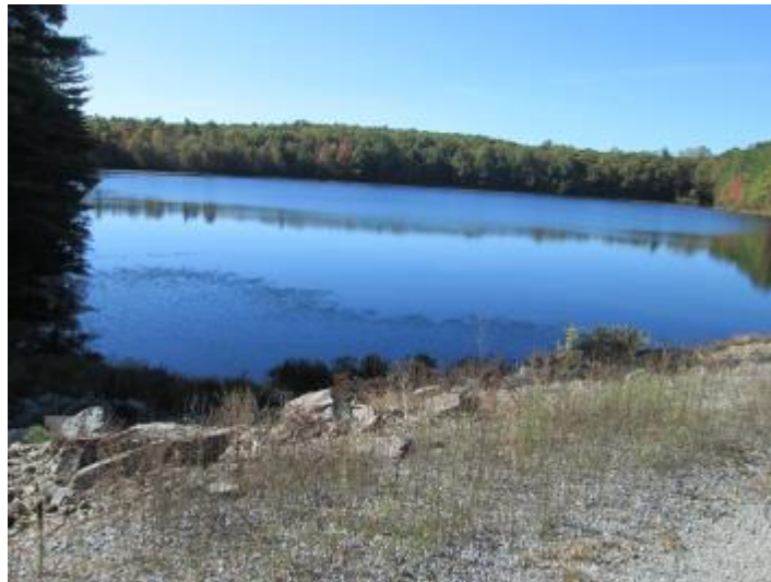
Figure 3.1.2.5.16: Carbaugh Run Dam Entrapment Area
