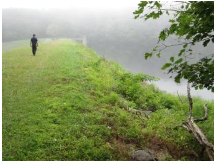
Figure 3.1.2.5.14: Antietam Dam Wall
