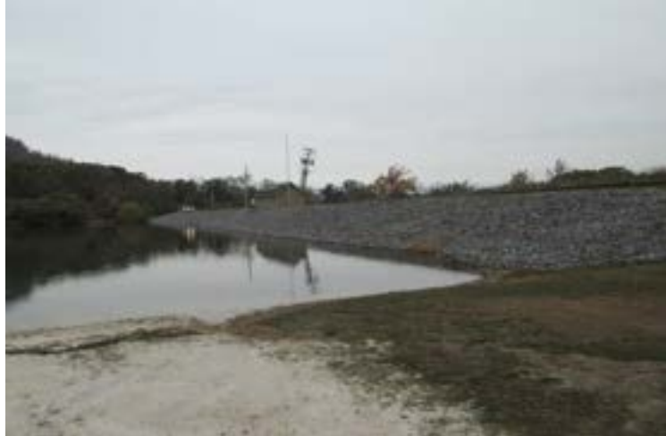
Figure 3.1.2.5.10: Whitetail – A Dam Wall
