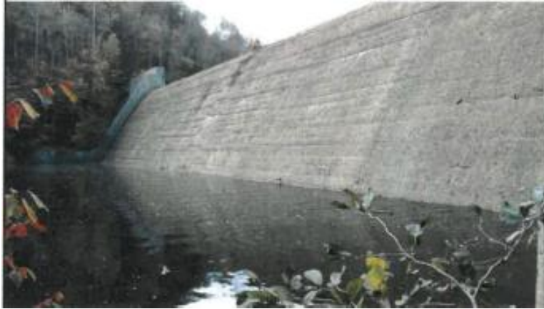
Figure 3.1.2.5.4: South Wall of Roxbury Dam
