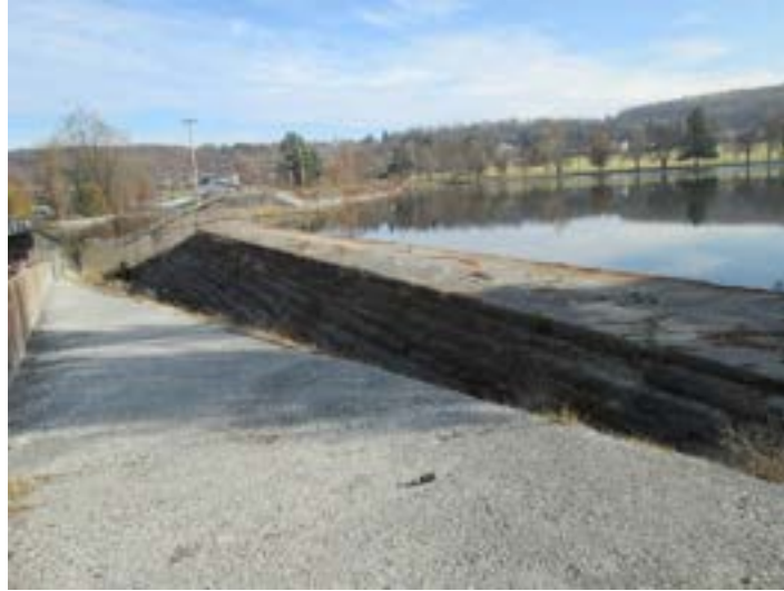
Figure 3.1.2.5.29: Lower Lake Royer Dam Spillway
