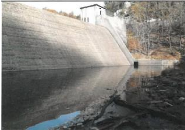
Figure 4.3.4.5.5: North Wing Wall of Roxbury Dam
