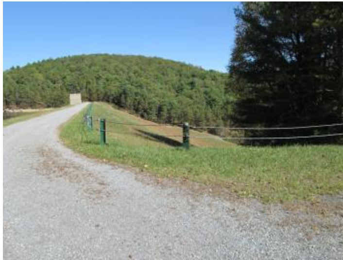
Figure 4.3.4.5.22: Long Pine Run Dam Wall
