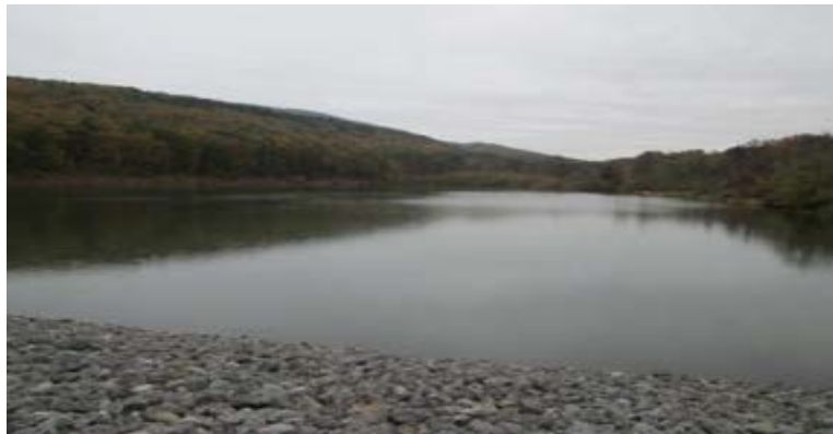
Figure 4.3.4.5.8: Whitetail Land Co. – A Dam Entrapment Area
