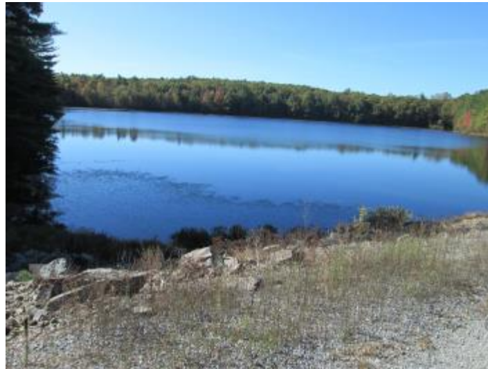
Figure 4.3.4.5.16: Carbaugh Run Dam Entrapment Area
