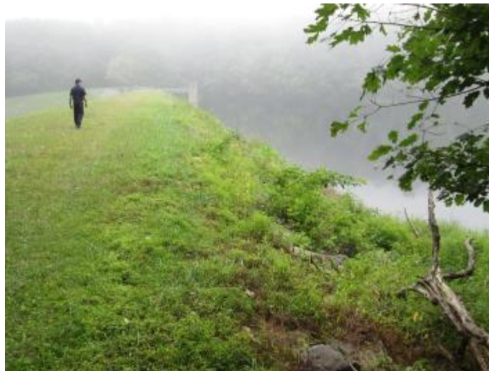
Figure 4.3.4.5.14: Antietam Dam Wall
