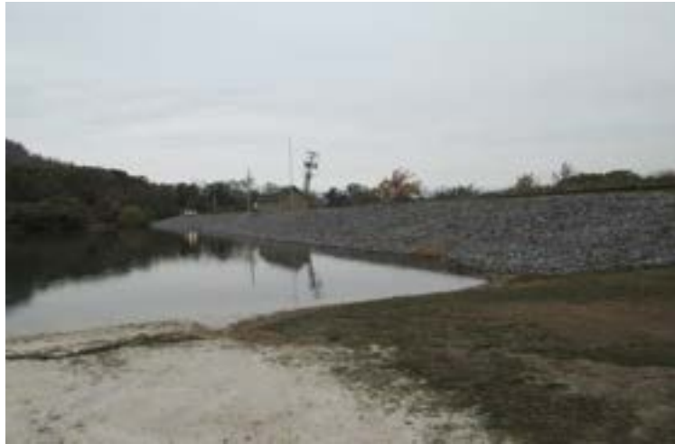
Figure 4.3.4.5.10: Whitetail Land Co. – A Dam Wall
