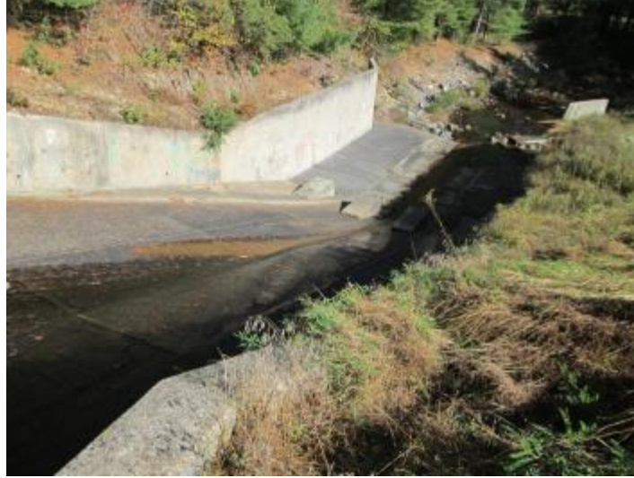
Figure 4.3.4.5.17: Carbaugh Run Dam Spillway
