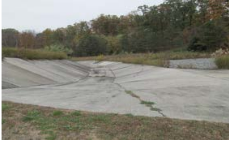
Figure 4.3.4.5.9: Whitetail Land Co. – A Dam Spillway
