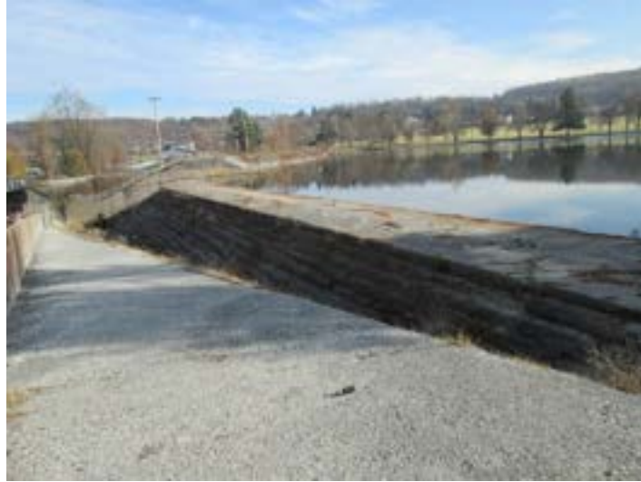
Figure 4.3.4.5.29: Lower Lake Royer Dam Spillway
