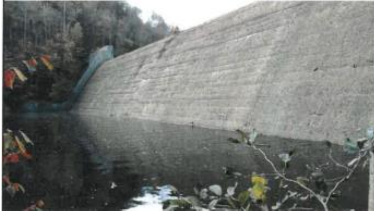
Figure 4.3.4.5.4: South Wall of Roxbury Dam
