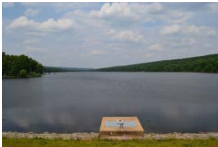
Figure 4.3.4.5.24: Meadow Grounds Dam Entrapment Area
