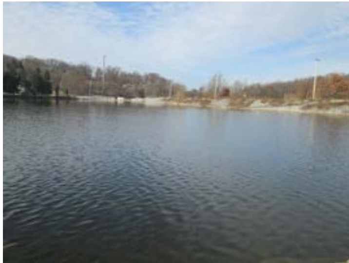
Figure 4.3.4.5.30: Lower Lake Royer Dam Wall
