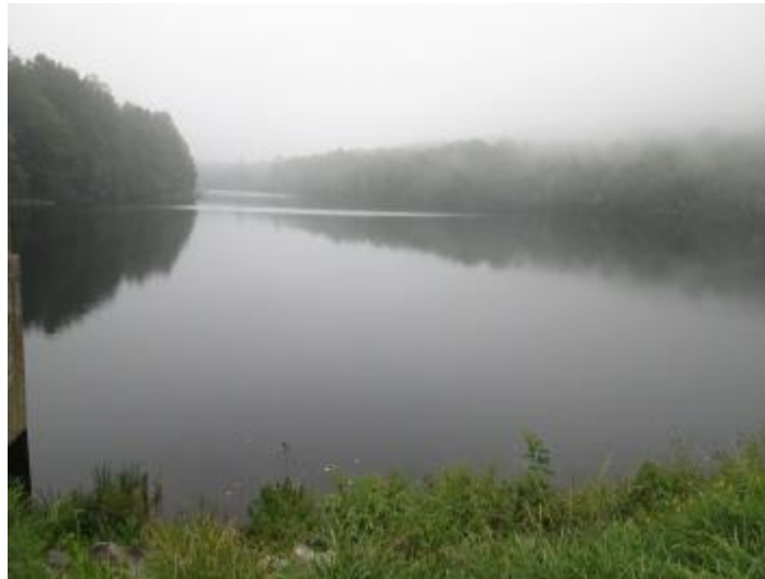
Figure 4.3.4.5.12: Antietam Dam Entrapment Area
