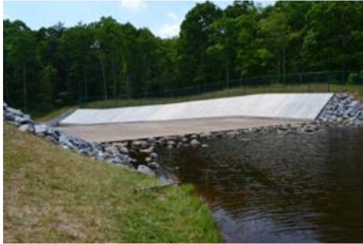
Figure 4.3.4.5.25: Meadow Grounds Dam Spillway
