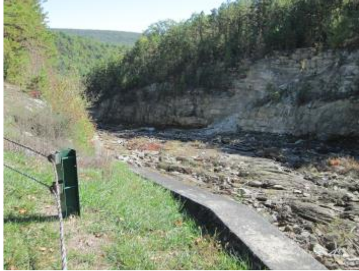
Figure 4.3.4.5.21: Long Pine Run Dam Spillway
