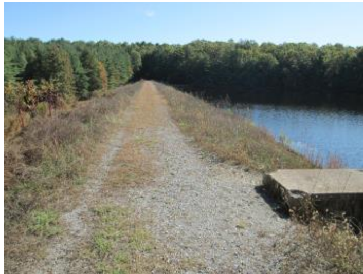
Figure 4.3.4.5.18: Carbaugh Run Dam Wall
