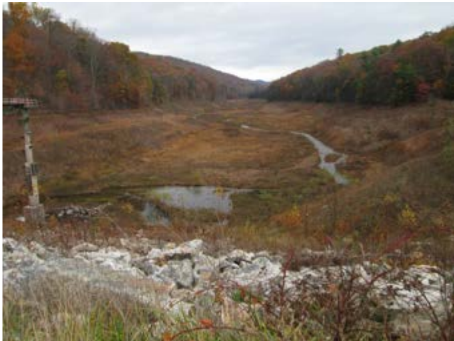
Figure 4.3.4.5.1: Gunter Valley Dam Lakebed
